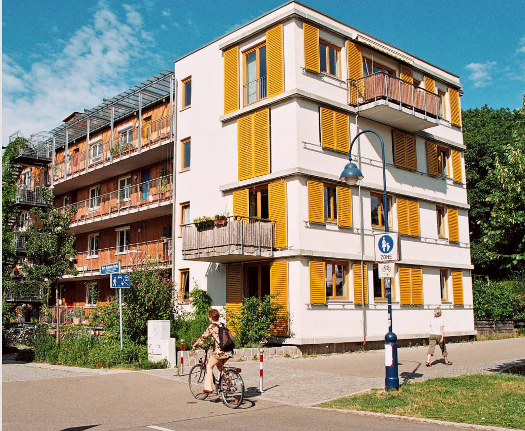
1 Distinctive architecture and car-free streets in Vauban
