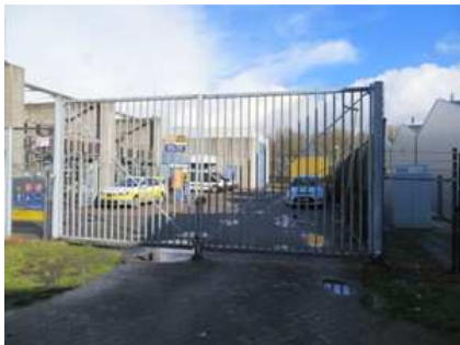
50/10 kV station (Transformatorstation)
